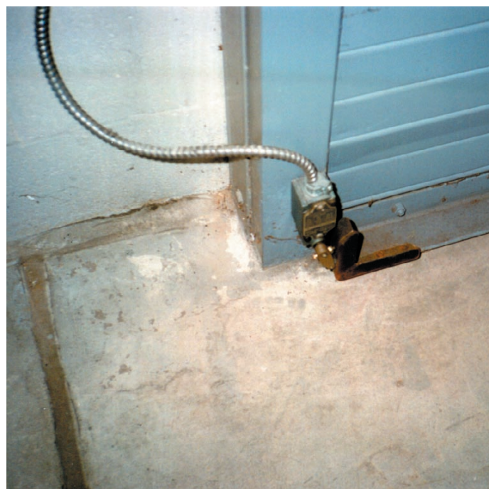
ROLLER TYPE DOOR SWITCH INSTALLED ON A ROLL-UP DOOR
